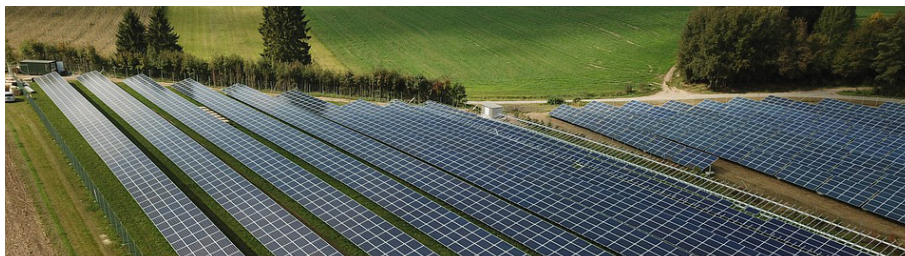
Figure 2: large PV power plant (Source: pixabay)
