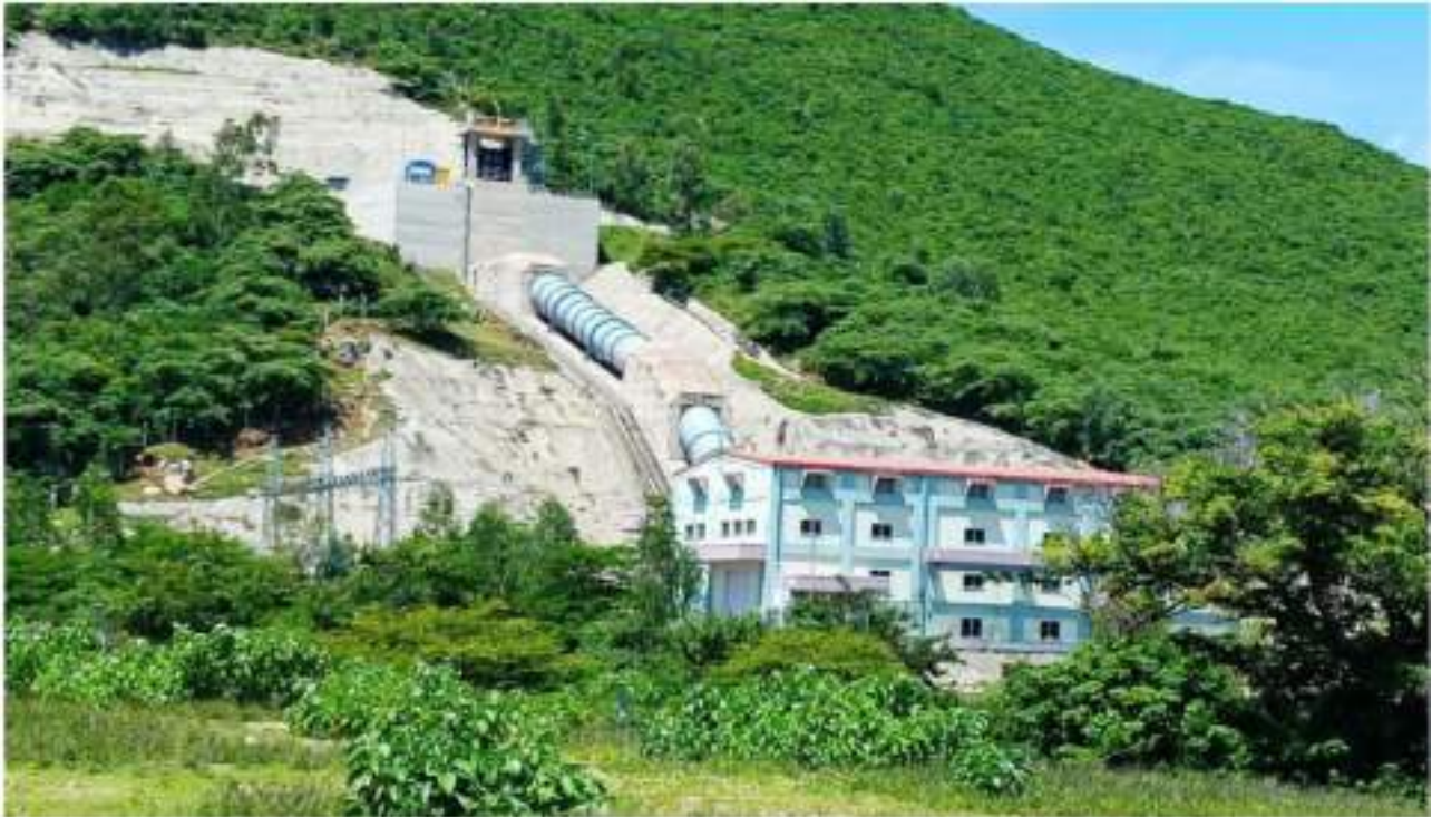
Figure 4-6 Sang'oro turbine (Sondu- Miriu hydro electric power station) (CIDP 2018)
