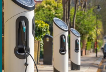
Figure 1: EV charging stations
