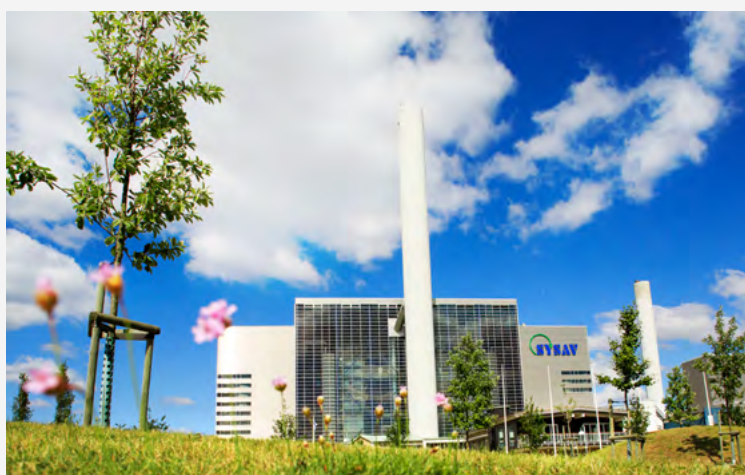
Figure 7. Sysav's waste cogeneration plant, Malmö. Source: Andreas Offesson © All rights reserved
