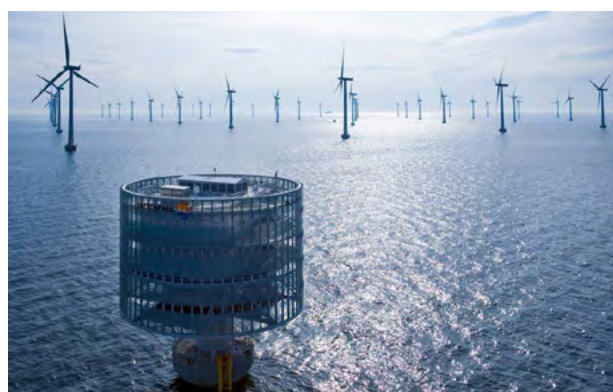
Figure 4: Siemens substation at the Lillgrund Wind Farm, Sweden. Source: (link)
