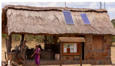
Figure 1: Solar home system in a village household set-up [11]
