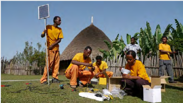
Figure 4: Solar Home Systems installation in Ethiopia. Source: International River [13]
