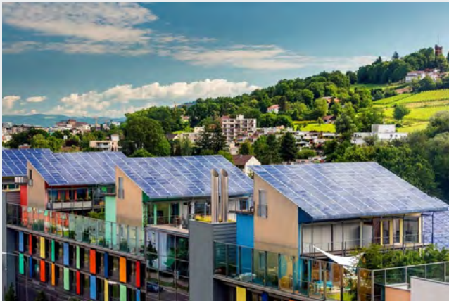
Figure 2: SPV Rooftop Systems Installed in Vauban, Freiburg. Source
