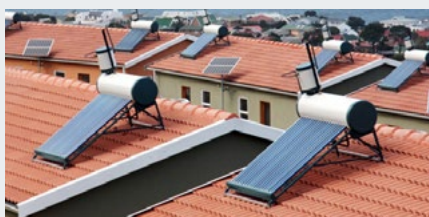
Figure 3: Evacuated tube collector (ETC)
