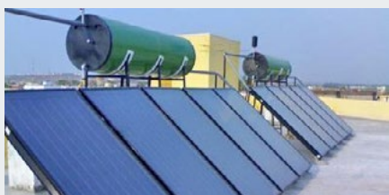
Figure 2: Solar flat plate collectors (FPC)
