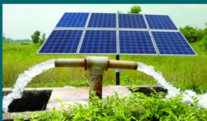
Figure 1: Solar Water Pump in Uganda [1]
