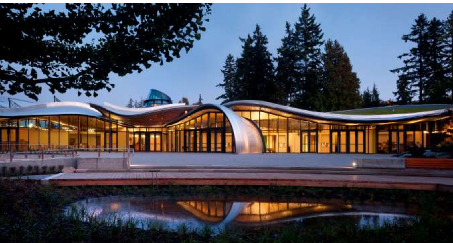
Figure 5: Vancouver's VanDusen Botanical Garden Visitor Center, an LEED Platinum building, completed in 2011. Source: City of Vancouver ( link )
