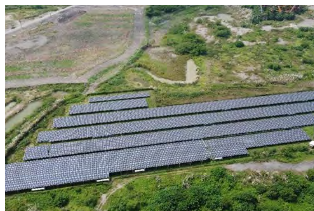
Figure 6. Gaoshu PV Demonstration Project. ©Pingtung County Government
