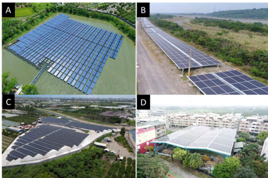
Figure 8. Methods of combined use of solar PV capacity for various types of land. Source: (Pan, Lu, & Yen, 2022)
