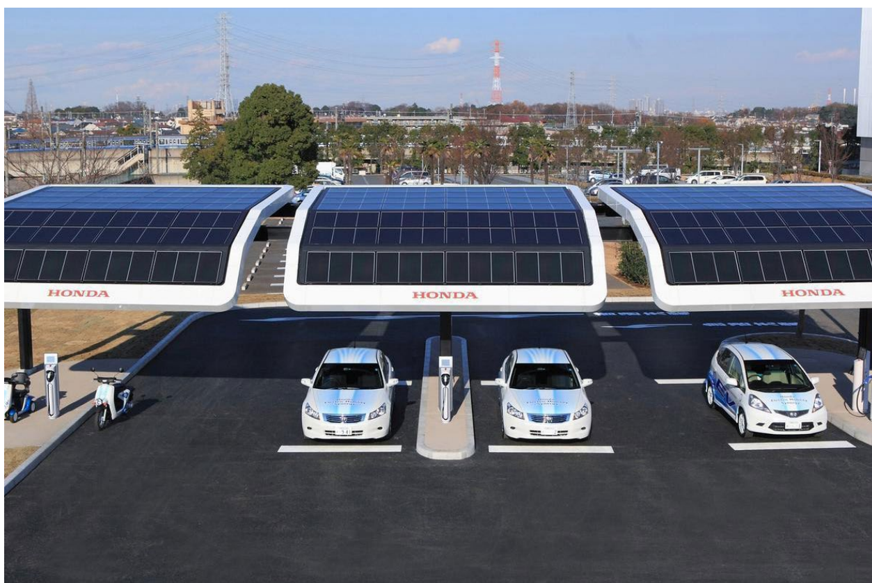
Figure 1: Honda's solar-powered public EV charging station. Source: New Atlas
