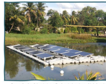
Source: A solar pilot project on a flood control water pond in Indonesia. Credit: Credit: Tommaso Scudato
