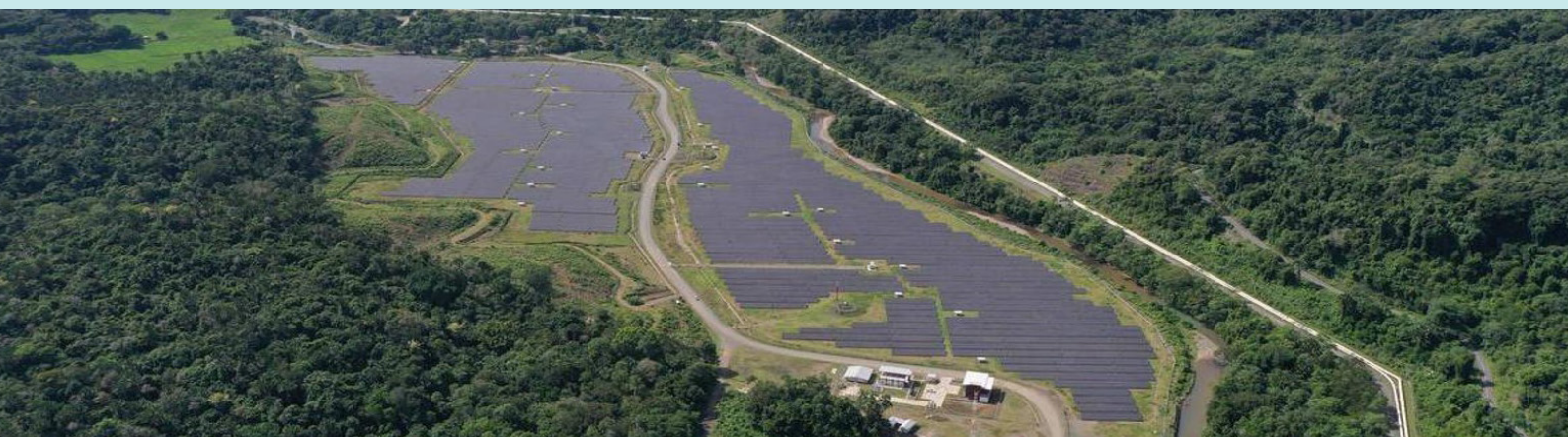
Figure 10. Constructed in 2021, the Amman Mineral Solar Power Plant (26 MWp) supplies about 20% of the electricity required for the AMNT smelter and processing unit in WNT. Source: DESDM NTB
