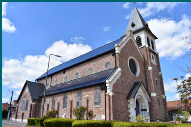
Source: Solar PV on the Church Roof - Loos-en-Gohelle
